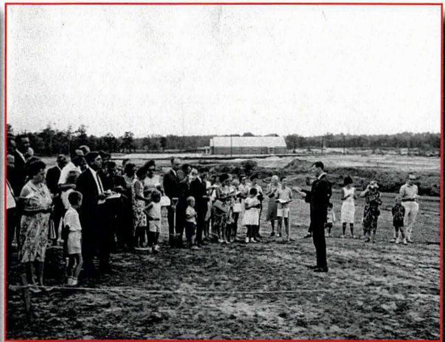
Groundbreaking. Notice St. Pius Catholic Church in the background.
